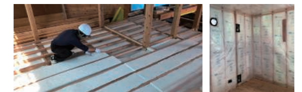
Installation of insulation on the floor, walls, and ceiling
