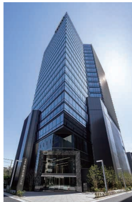
Sumitomo Fudosan Shinjuku Minamiguchi Building (Completion: Mar 2024) Shibuya Ward, Tokyo No. of floors: 17 above / 1 below ground Gross floor area: 23,874 m 2
