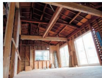
Interior stripped down to its main frame
