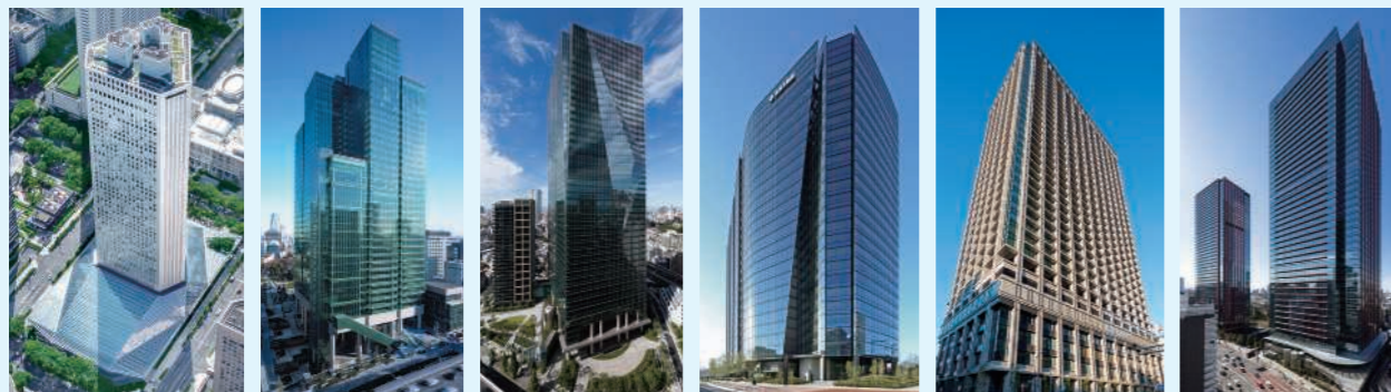
Shinjuku Sumitomo Building, Izumi Garden Tower, Sumitomo Fudosan Roppongi Grand Tower, Sumitomo Fudosan Osaki Garden Tower, Tokyo Nihombashi Tower, Sumitomo Fudosan Tokyo Mita Garden Tower
