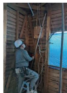
Seismic reinforcement work
