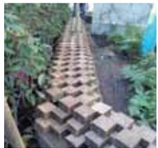
We have developed technology for reusing soil from condominium construction sites to create blocks with few CO<sub>2</sub> emissions. The blocks are environmentally friendly because they are made of natural materials, which will eventually return to the ground at the end of their life. The blocks are used in planted zones in condominium sites.
