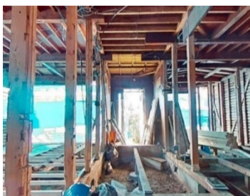
Structural frame being reused
