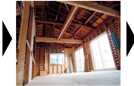
During renovation work (Interior stripped down to its main frame)
