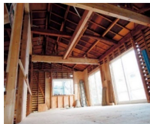
Interior stripped down to its main frame
